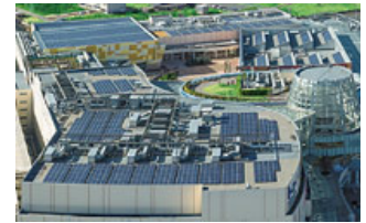
Rooftop solar panels at LaLaport KASHIWANOHA
