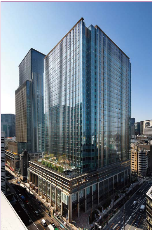
▶ Nihonbashi Muromachi Mitsui Tower (Chuo-ku, Tokyo)
