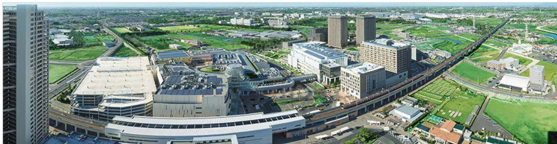
Kashiwa-no-ha Smart City and Kashiwanoha-campus Station
