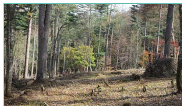
▶ Ground clearing complete
