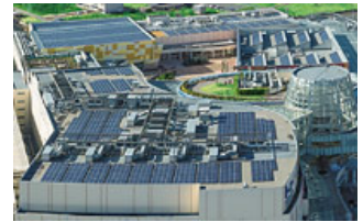
Rooftop solar panels at LaLaport KASHIWANOHA
