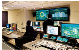
Kashiwa-no-ha Smart Center monitors regional energy supply and demand
