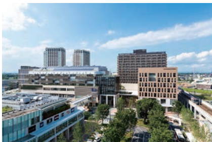
Kashiwa-no-ha Smart City is a model for the next-generation environmental cities of the future
