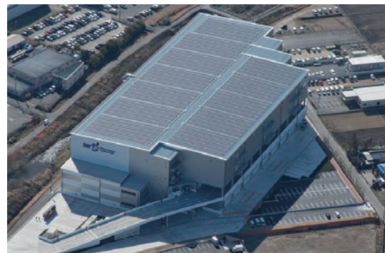
Solar power panels at MFLP Komaki
