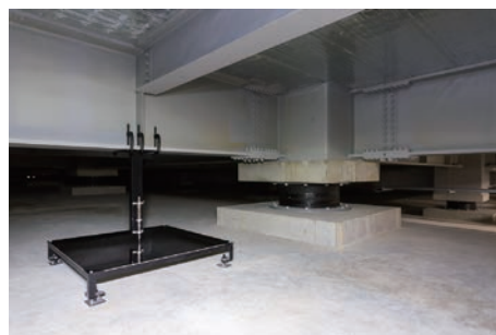
MFLP Hino seismic isolation pit
