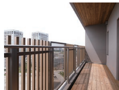
In balcony ceiling and flooring materials in "Park Axis Kashiwa-no-ha" rental residences
