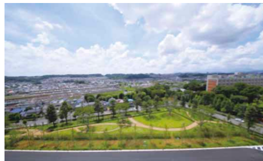
Open spaces and promenades located along the southern end of the MFLP Hino site.
