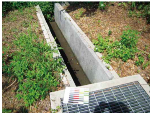
Use of environmental activation concrete at a drainage ditch
