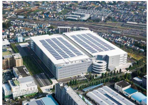
Solar panels at MFLP Hino
