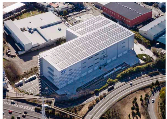
Solar panels at MFLP Kashiwa
