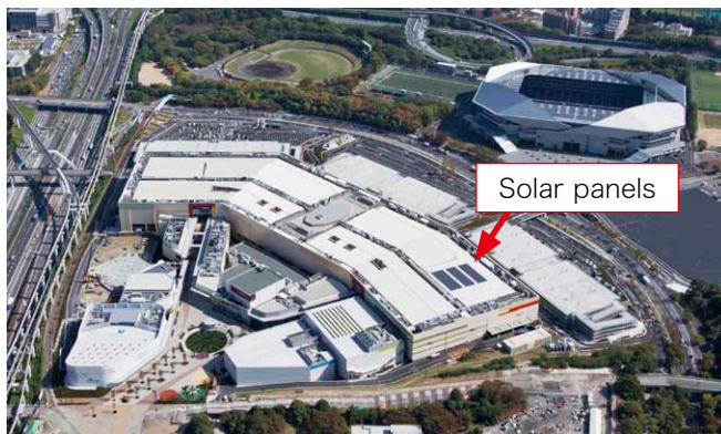
EXPOCITY's solar panels (photographer: SS Osaka Co., Ltd.)
