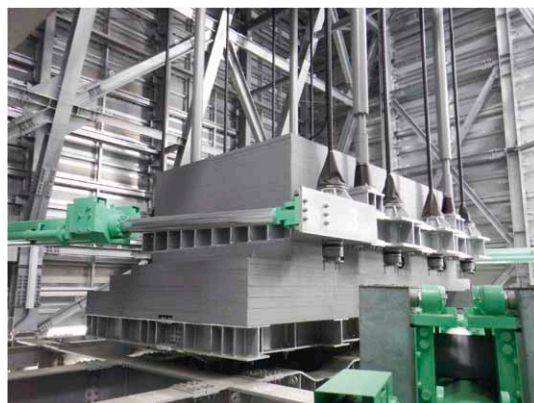
TMD internal structure
