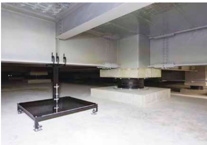
Anti-seismic structure (MFLP Hino)
