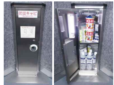
Cabinets that store emergency supplies (MFLP Hino)
