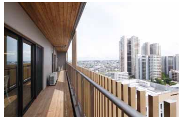
In balcony roof and flooring materials
