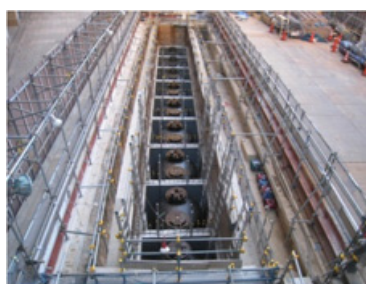
Oil tank expansion work (Kasumigaseki Building)
