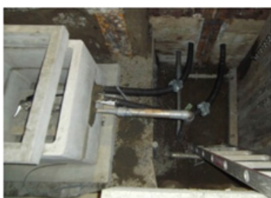
Well tunneling work (Nihonbashi Mitsui Tower)
