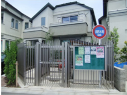
Water tank site for firefighting
