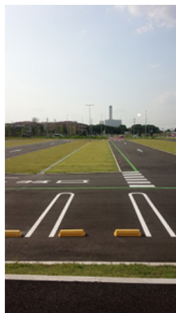
Grassy sections installed at parking lots
