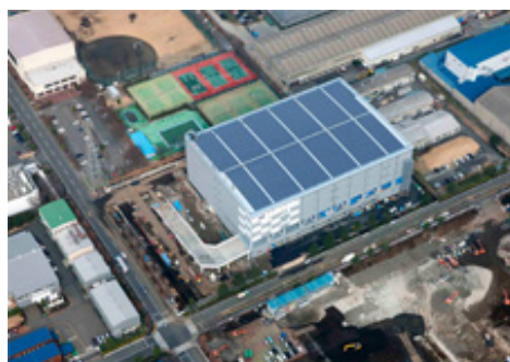
Solar panels on the roof of MFLP Atsugi
