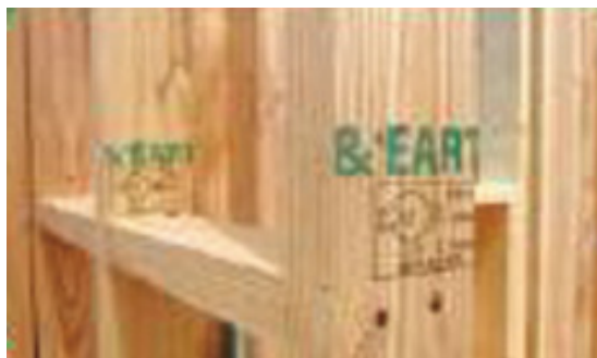
Plywood for structure of detached housing
