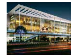
Lianhua Road Station Building Retail Facilities
