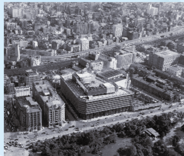
Before development The former Hibiya Mitsui Building
