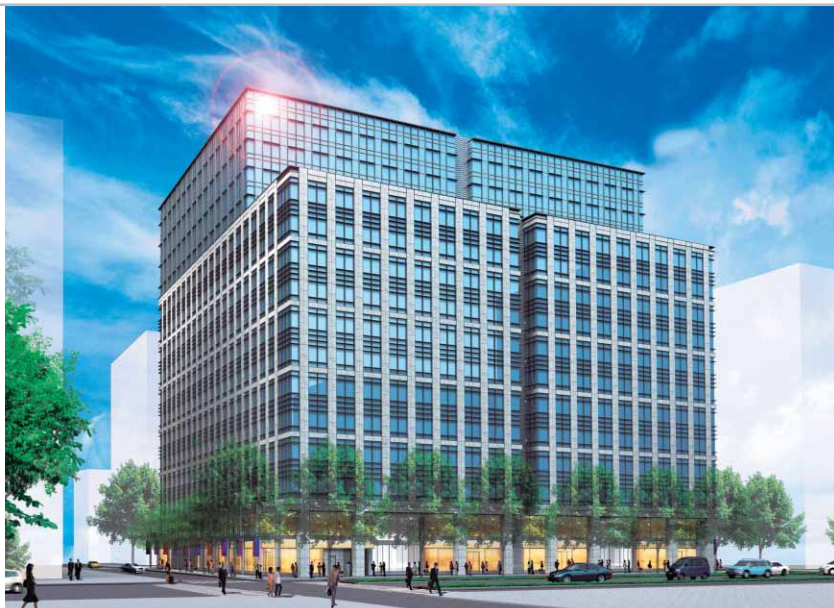
Yodoyabashi Redevelopment (Office building / Completion scheduled for March 2008 / 44,000m 2 )
