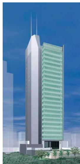
Kita Aoyama Project (Office building / Completion scheduled for August 2008 / 47,000m 2 )
