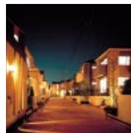
Fine Court Ogikubo Masters Fort (Completed in May 2002/ 13 units)
